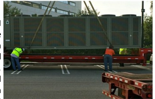
Figure 2: Partnership II air-cooled chillers arriving and being crane-lifted to the rooftop
